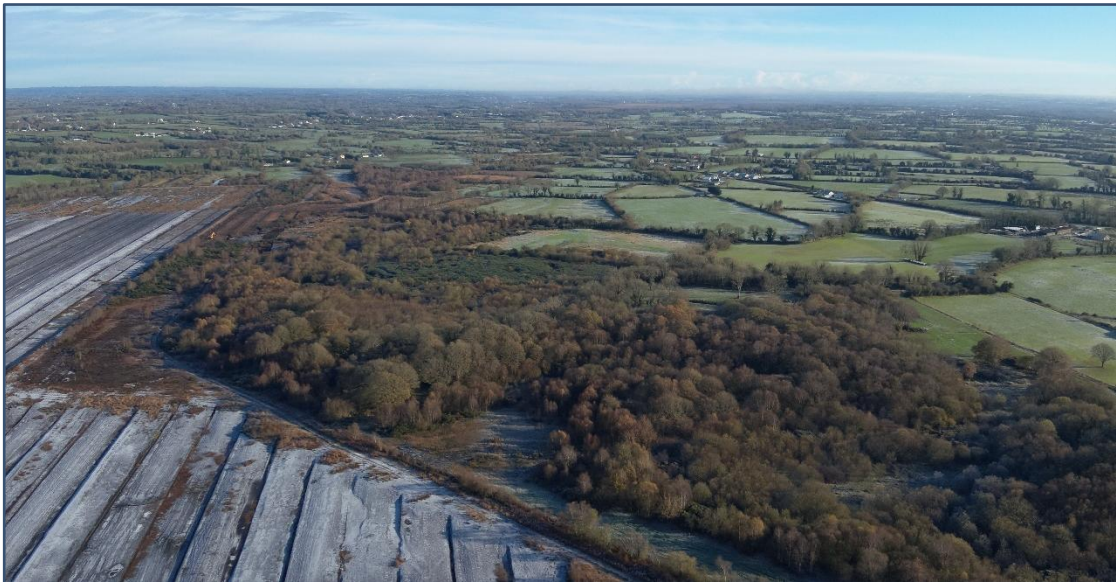
Plate 14-25 Drone Image for Landscape Context: Views east of the Proposed Wind Farm of a large pocket of woodland
