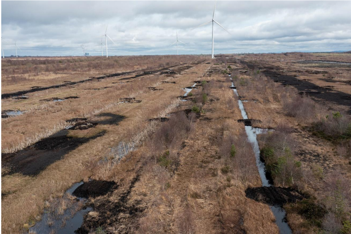
Plate 11-1 Peatland rehabilitation implemented in the form of drain blocking proximal to wind farm infrastructure at Cloncreen Wind Farm.
