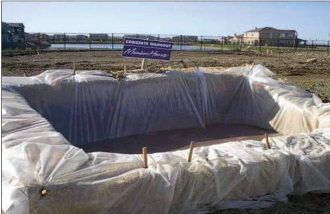
Plate 4-4 Concrete washout area
