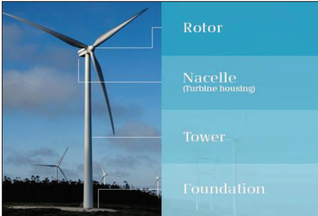
Plate 4-1 Wind Turbine Components
