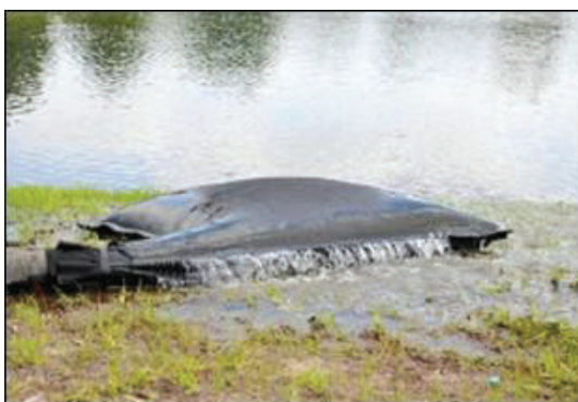
Plate 4-7 Silt Bag with water being pumped through
