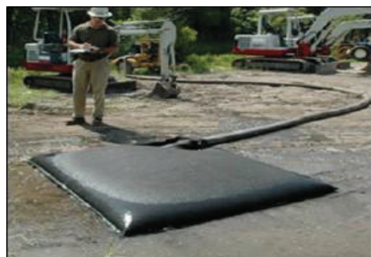
Plate 4-8 Silt bag under inspection
