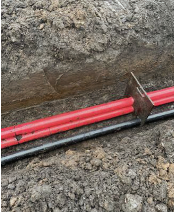
Plate 4-11 Typical Cable Trench View left, reinstated trench, right. Source: BnM.
