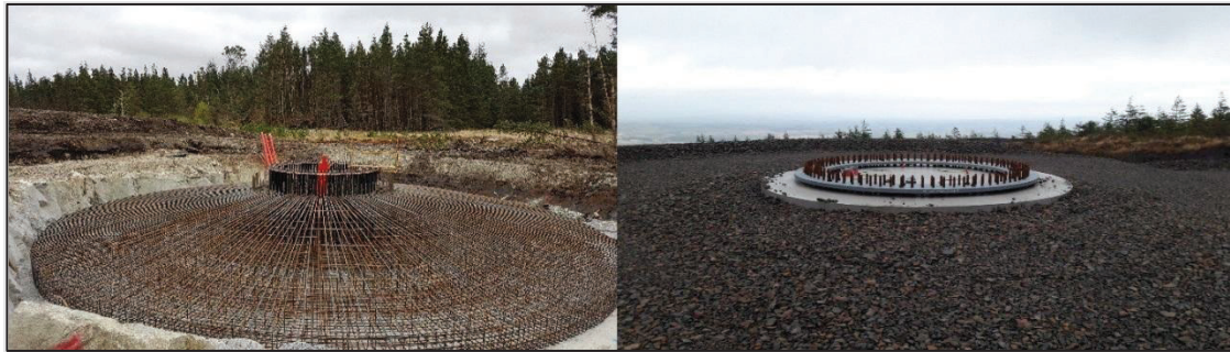
Plate 4-2 Turbine 'Anchor Cage' and finished turbine base
