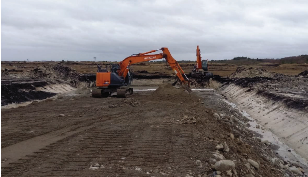
Plate 4-9 Internal roads under construction using the excavate and replace method. Source BnM.
