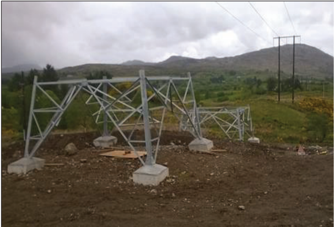
Plate 4-14 Steel lattice tower foundation complete. Source: BnM
