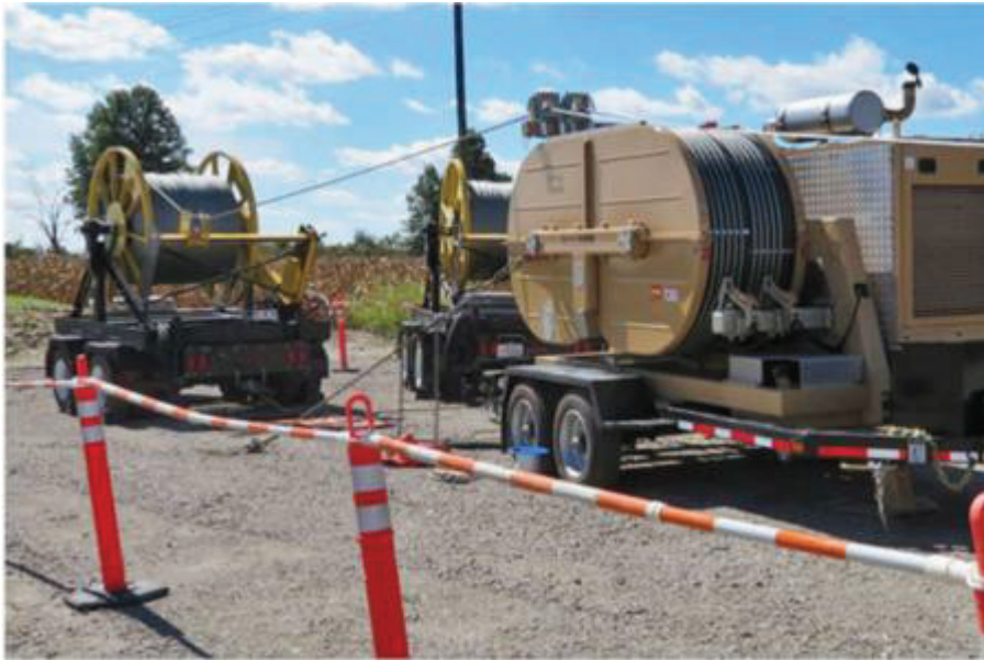
Plate 4-17 Puller – Tensioner Machine. Source: BnM
