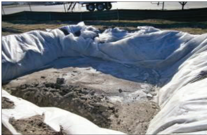
Plate 4-5 Concrete Wash Out Area
