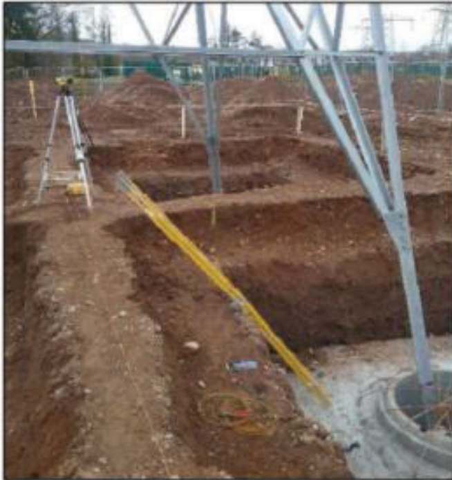
Plate 4-12 Steep Back Excavation. Source: BnM
