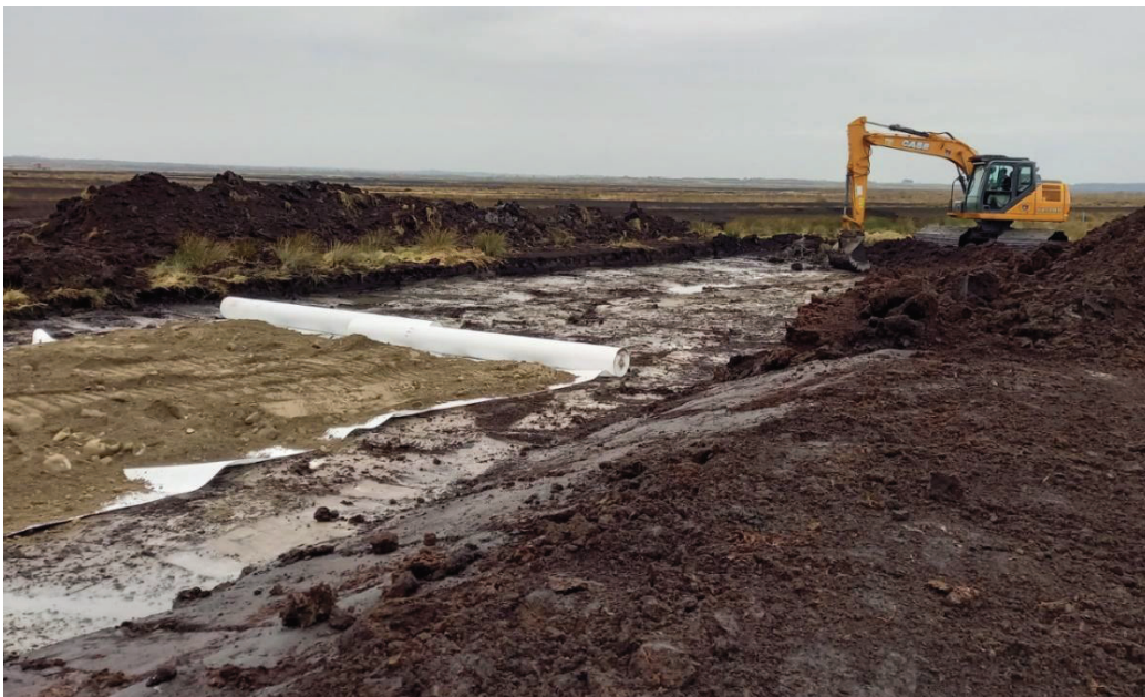
Plate 4-10 Internal Road under construction demonstrating laying of geogrid/geotextile. Source BnM.
