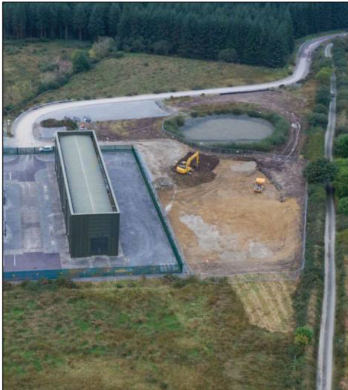
Plate 4-18 Typical 220kV GIS Switching Substation. Source: BnM
