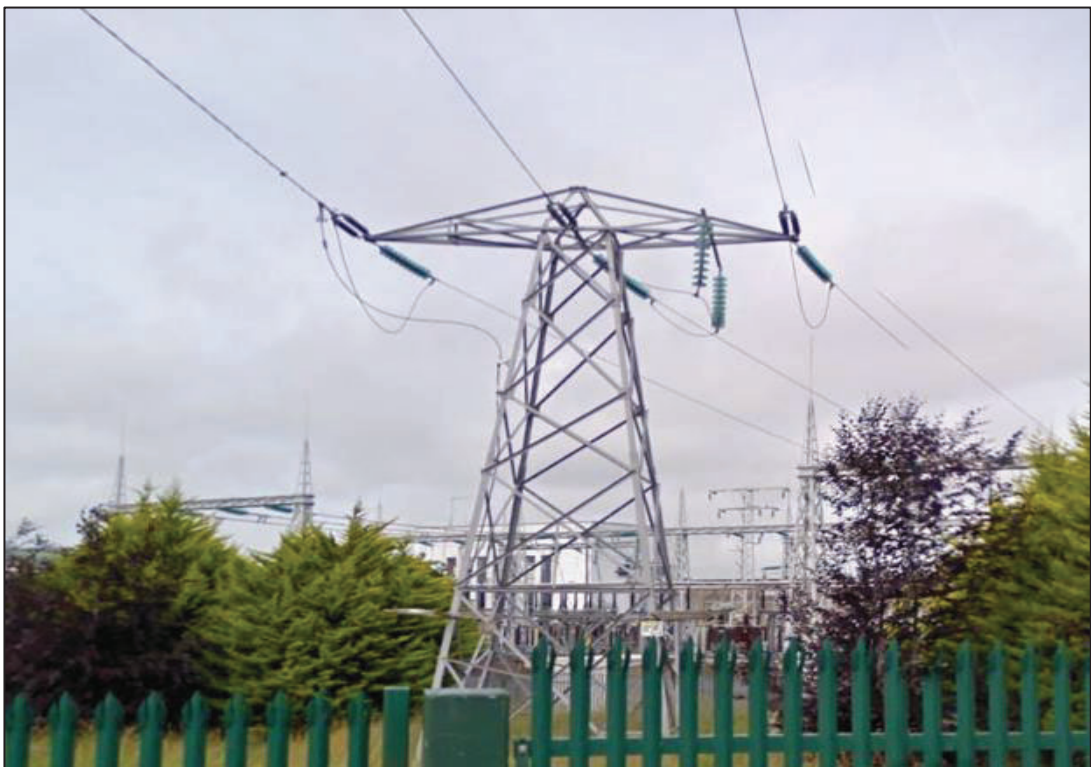
Plate 4-15 Completed End Mast Tower. Source: BnM
