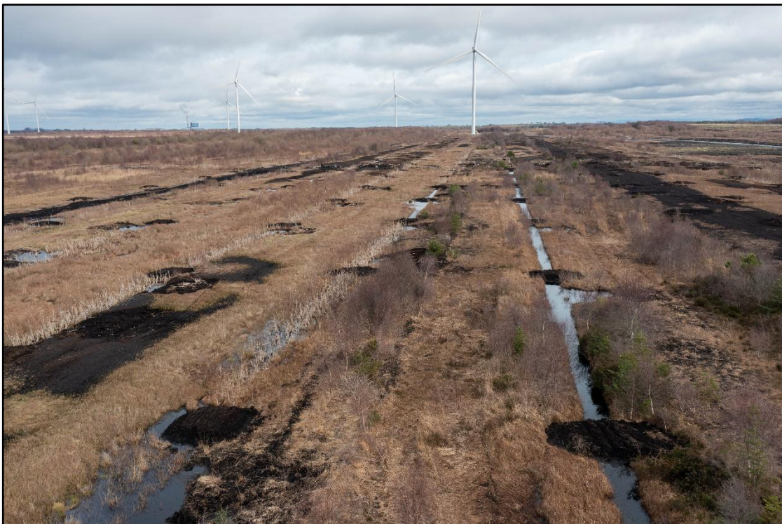
Plate 2-2 Peat dams installed on cutover bog within the Cloncreen windfarm site
