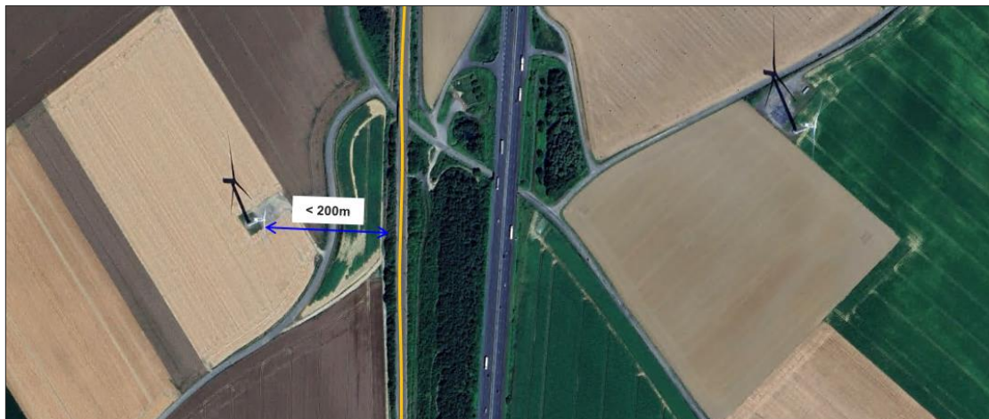
Figure 11. Example of existng wind tubrines near rail line
