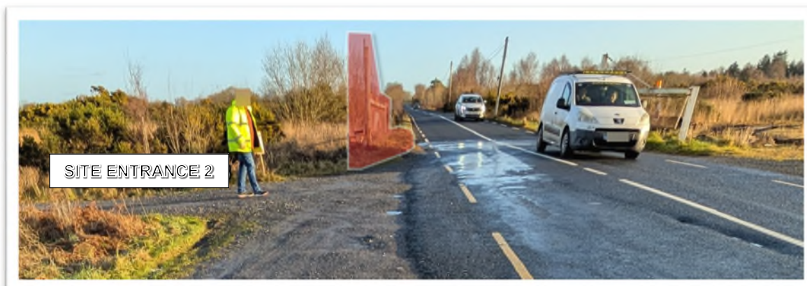
Figure 2.2 – Drivers Exiting from Access – View to Left Obscured by Level Crossing Gate
