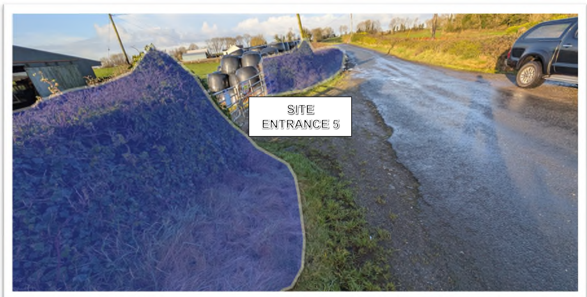
Figure 2.4 – Visibility Splays Partially Obscured in Both Directions at Site Entrance 5
