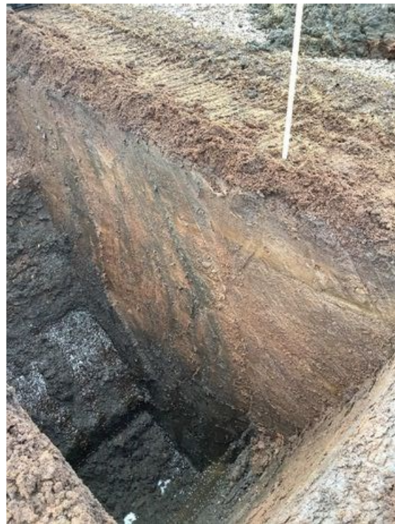
Plate 6: TP3 after peat excavation
