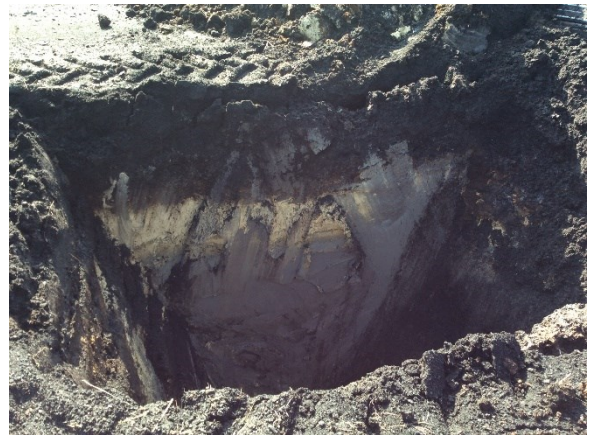
Plate 28: TP12a Post excavation
