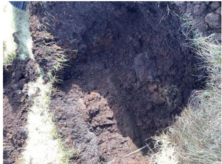
Plate 42: TP21 showing peat collapse
