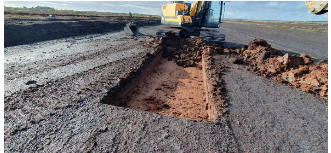
Plate 2: Stripping of TPCC003 at northwest of site, facing southwest
