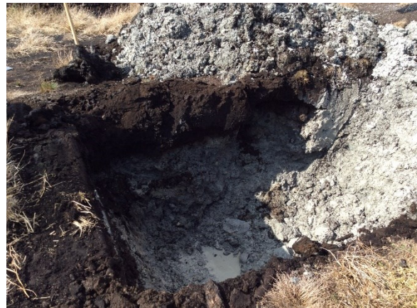
Plate 20: TP9 after excavation
