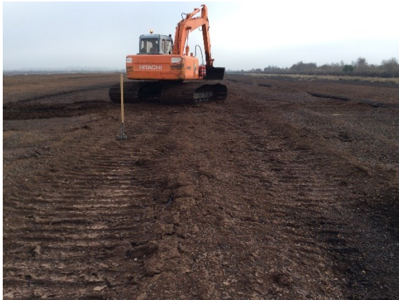
Plate 15: TP7a prior to excavation
