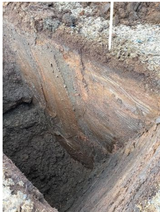
Plate 12: TP6 after peat excavation
