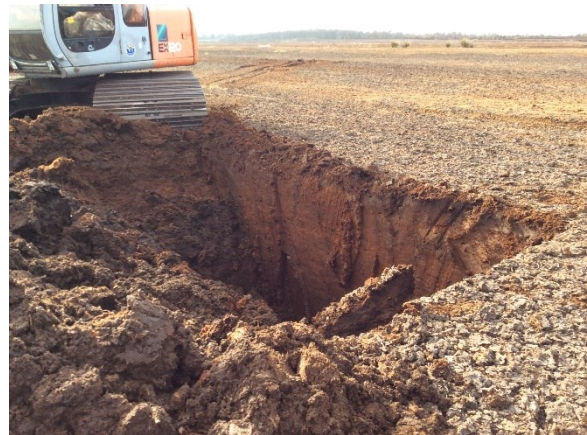
Plate 38: TP15 after excavation
