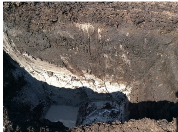
Plate 4: TP2 after excavation
