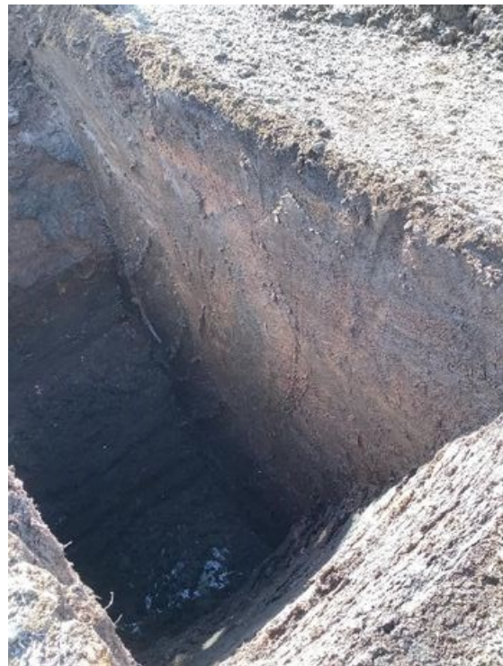
Plate 44: TP22 after peat excavation
