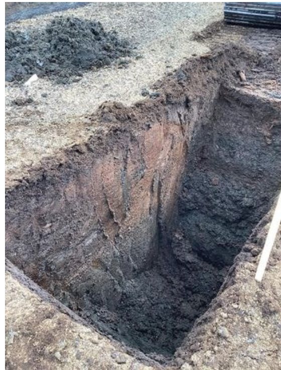
Plate 18: TP9 after peat excavation
