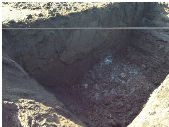
Plate 30: TP12B after excavation
