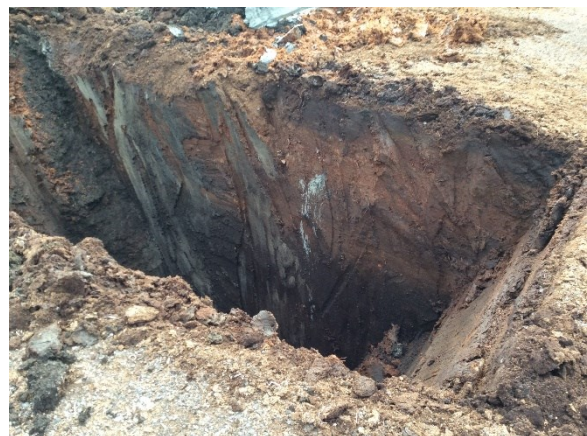
Plate 14: TP7 after excavation
