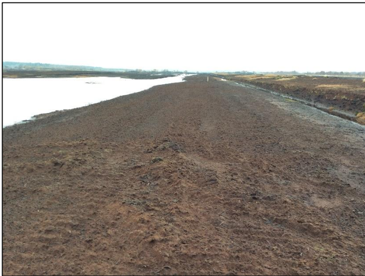
Plate 2: Hardstand for T1, looking NE.
