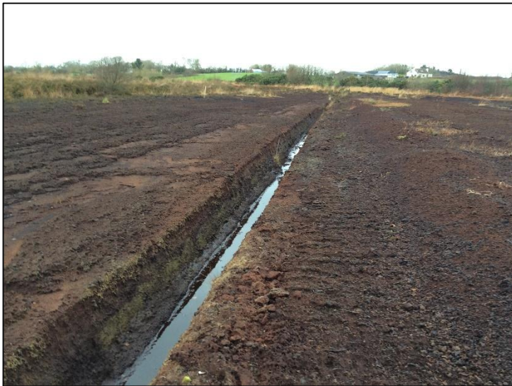
Plate 49: Proposed tower hardstand, looking NW.
