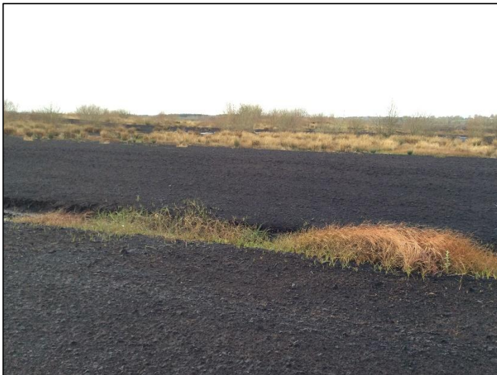
Plate 20: Hardstand for T9, looking SW.
