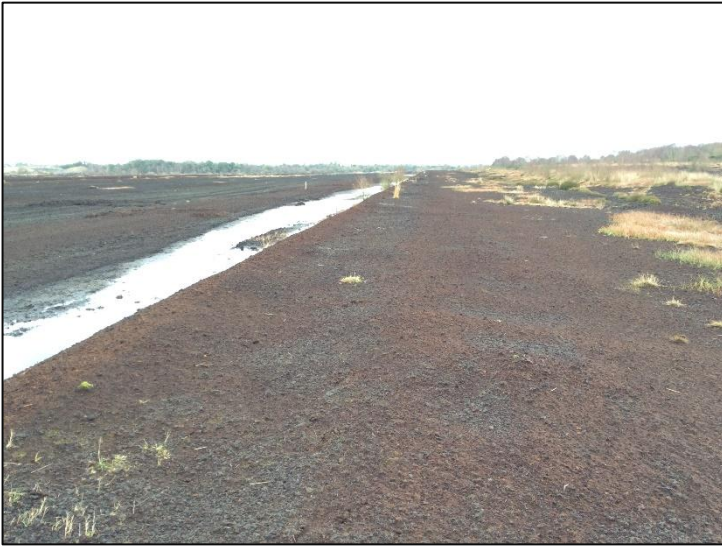
Plate 31: Hardstand for T15, looking NE.
