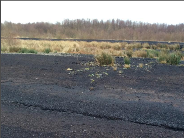
Plate 3: General location of T2, looking SE.
