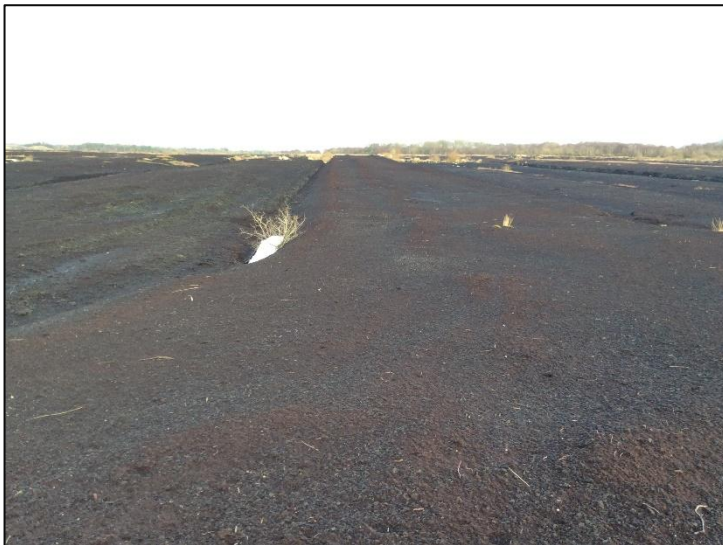
Plate 35: Temporary construction compound SW of T15, looking NE.
