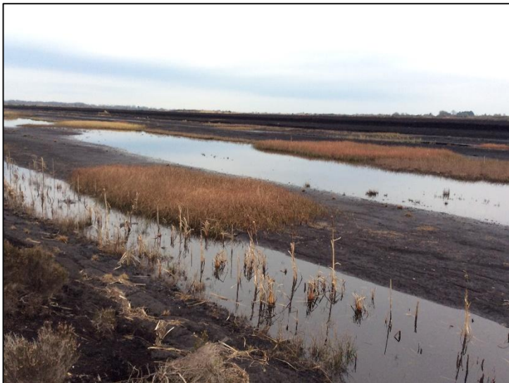
Plate 11: Hardstand for T6, looking SE.
