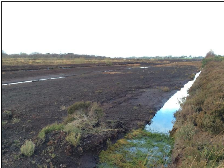
Plate 44: Proposed road from onsite substation, looking NW.
