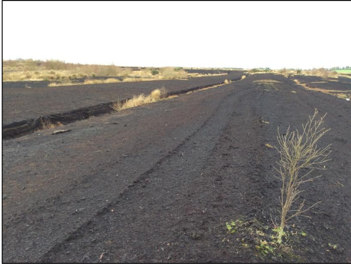
Plate 21: Hardstand for T10, looking N.
