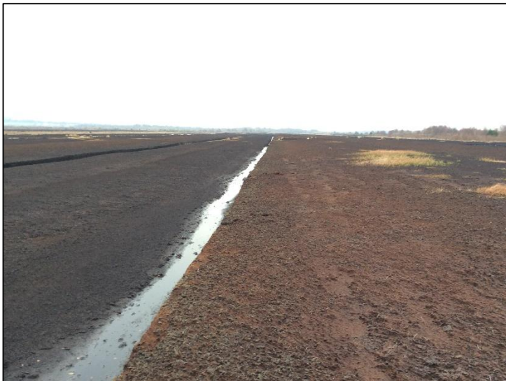
Plate 14: Hardstand for T7, looking NE.
