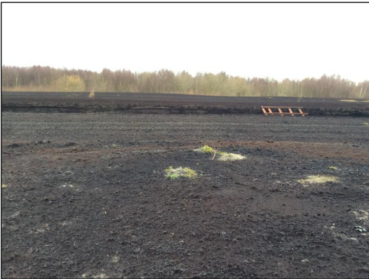
Plate 4: Hardstand for T3, looking NW.
