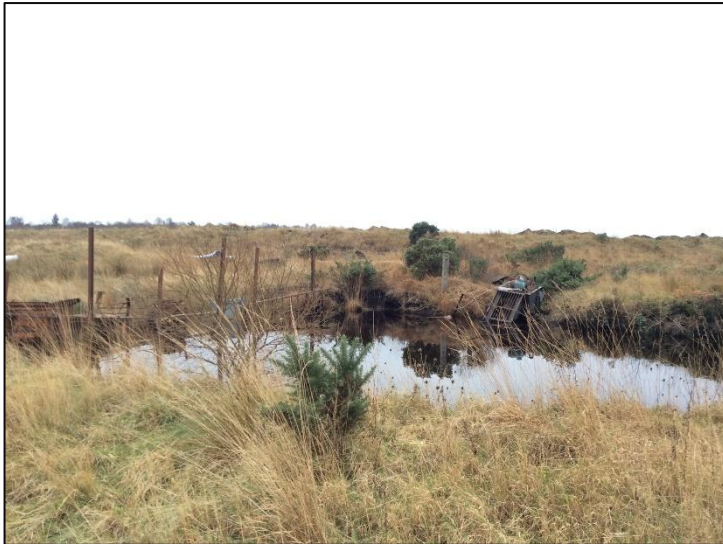
Plate 57: Proposed pump station, looking SW.
