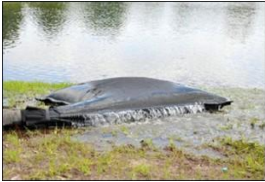
Plate 2-1 Silt Bay with water being pumped through
