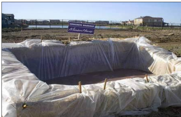
Plate 3-1 Concrete washout area
