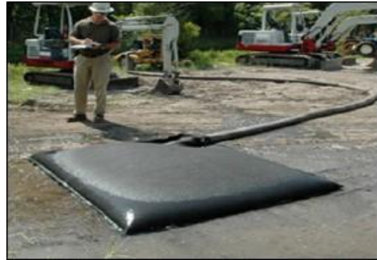
Plate 2-2 Silt Bay under inspection
