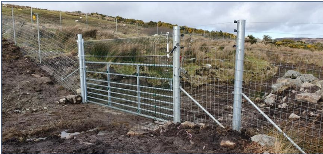
Plate 3- 2 Example predator-proof fencing and access gate broadly in-line with proposed specifications (for illustrative purposes only. source - as per above).
