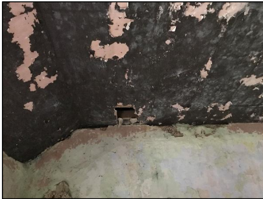
Plate 3-3 Interior of house showing potential access to the attic
