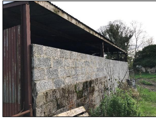
Plate 4-7 Exterior of large shed showing external brick wall
