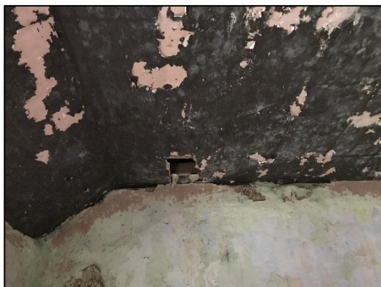
Plate 4-3 Interior of house showing potential access to the attic
