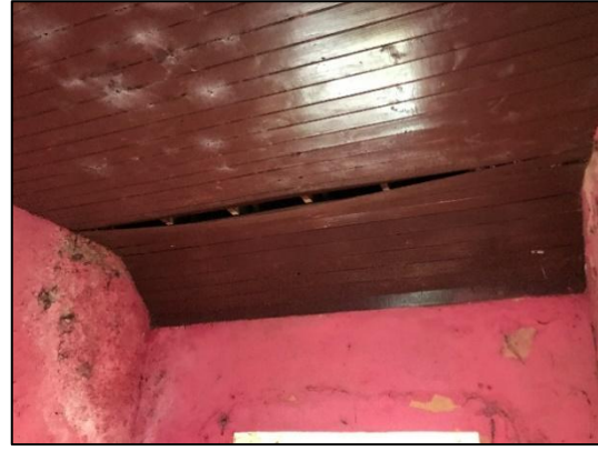
Plate 3-2 Interior of house showing potential access to the attic
