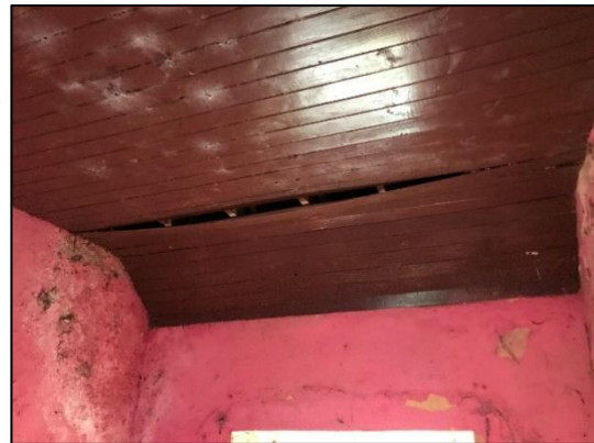
Plate 4-2 Interior of house showing potential access to the attic
