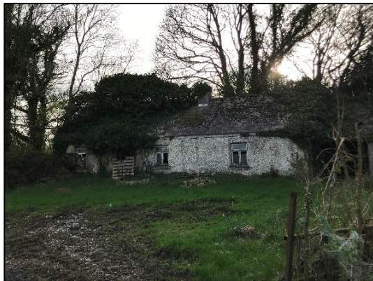
Plate 4-1 Exterior of house showing open windows and ivy overgrowth
