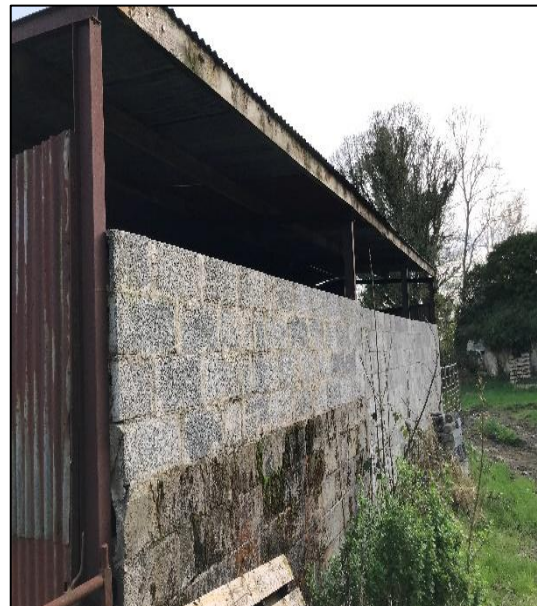
Plate 3-7 Exterior of large shed showing external brick wall
