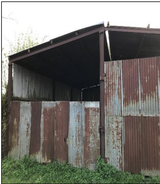
Plate 3-6 Shed Exterior showing galvanised walls and roof
