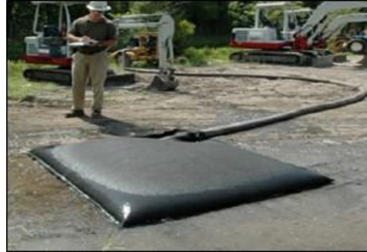
Plate 2-2 Silt Bay under inspection
