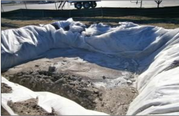
Plate 3-2 Concrete washout area
