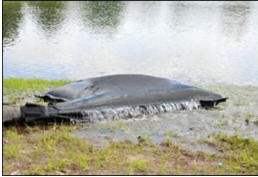
Plate 2-1 Silt Bay with water being pumped through
