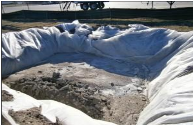
Plate 2 Concrete washout area
