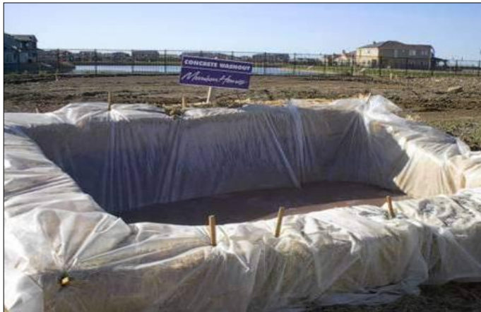
Plate 1 Concrete washout area
