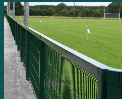
Ballyfore GAA - completed fence.
